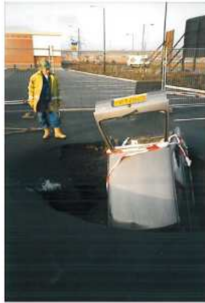
Figure 2.7: Shaft collapse in a car park.
