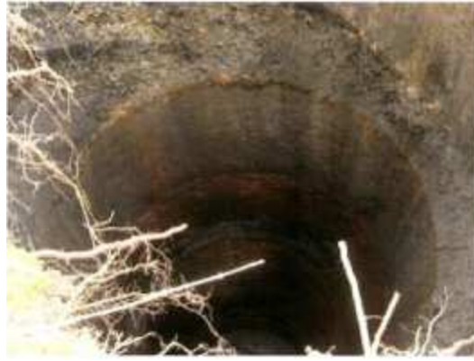
Figure 2.5: Collapse of Shaft in Lancashire, UK (Lecomte et al 2012)
