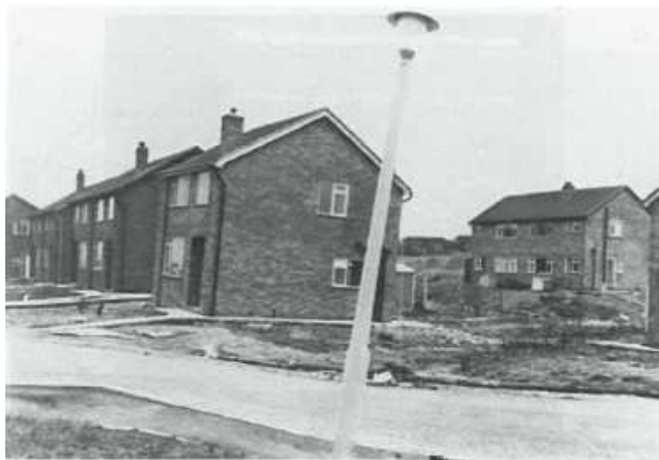
Figure 2.14: Tilt Subsidence due to longwall mining (Whittaker & Reddish, 1989)
