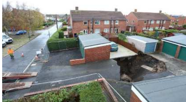
Figure 2.11: Initial collapse of Gosforth Shaft
