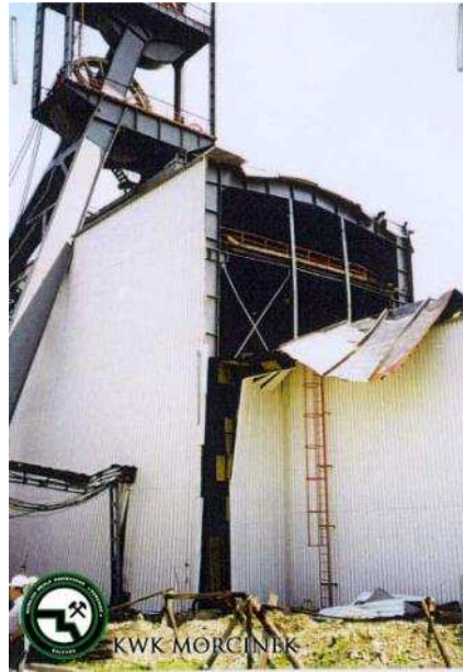
Figure 2.19: Effects of methane explosion in backfilled shaft III. Source: JSW S.A.’
