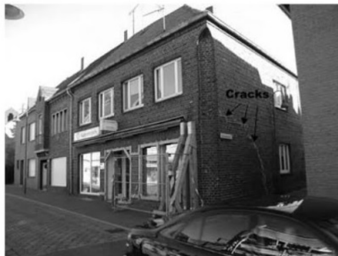
Figure 2.15: The building qualified for the total damage as a result of an irregular uplift of the ground surface
