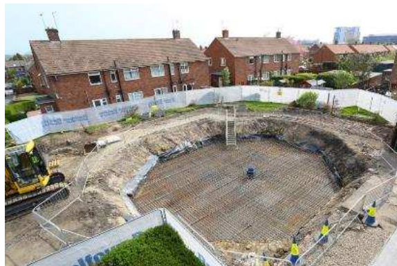
Figure 2.12: Construction of the hexagonal, steel reinforced concrete slab
