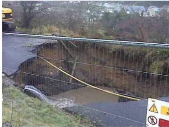
Figure 2.9: Collapse of Shaft at Tirphil.
