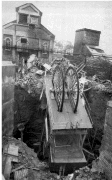
Figure 2.8: Collapse of Barony Colliery No 2 Shaft Lining (Lecomte et al, 2012)
