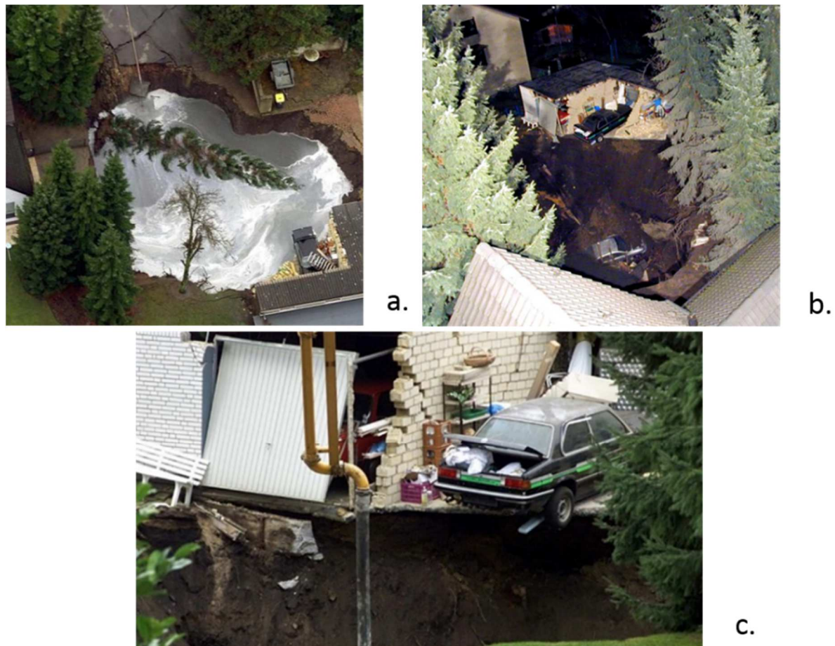
Figure 2.6: Sinkhole in residential development in the city of Bochum (a. (Nölkensmeier, 2000); b. (Seiler, 2016); c. (Rönsberg, 2012))
